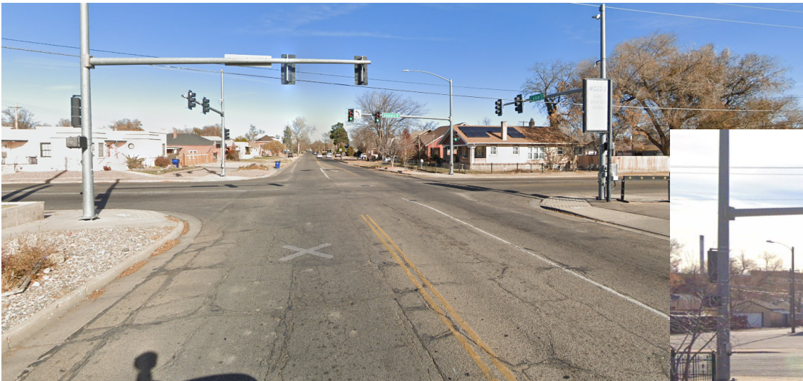
Lake Avenue, Northbound
