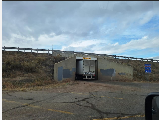
Photo 3 : Taken from east side of I-25a looking northbound. A WB-67 narrowly fitting into the existing box culvert heading west onto Purcell Blvd.
