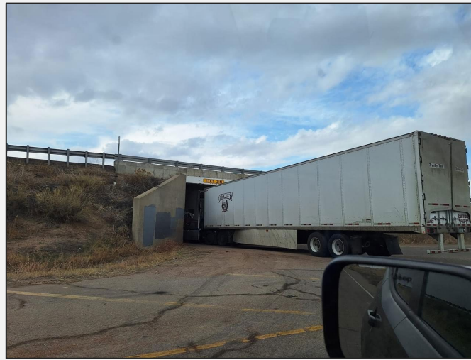
Photo 2 : Taken from east side of I-25a looking northbound. A WB-67 lining up to attempt driving through the existing single lane box culvert onto westbound Purcell Blvd.
