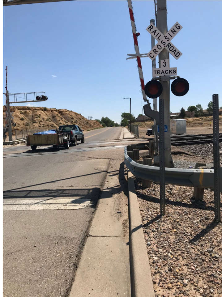
Missing sidewalk, ADA curb ramps, lack of bicycle infrastructure make this access point very dangerous inaccessible for the disabled community
