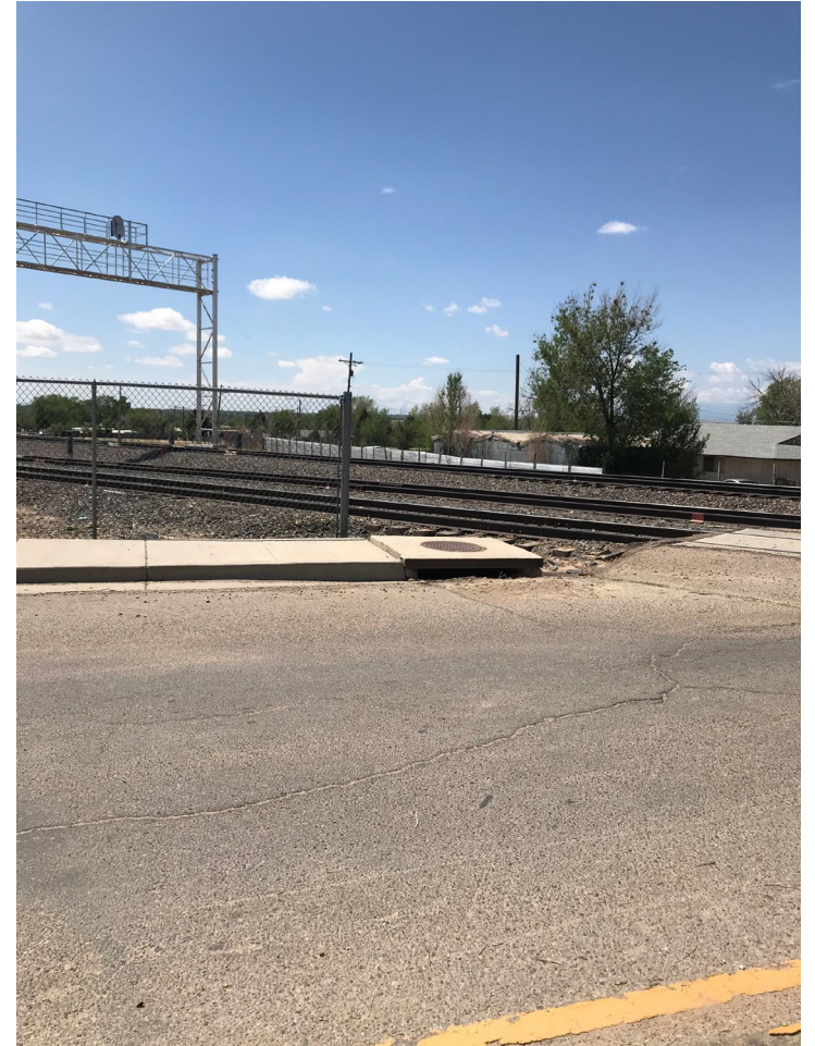
Missing sidewalk, ADA curb ramps, lack of bicycle infrastructure make this access point very dangerous inaccessible for the disabled community
